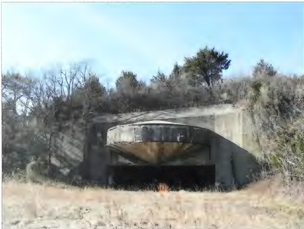
Figure 3.48. View looking southwest at emplacement #2, Battery Kingman. Designed to shield the gun platform from overhead fire, the concrete canopy exhibits efflorescence indicating water is infiltrating the concrete and drawing out impurities to the surface (Olmsted Center, January 2009).
